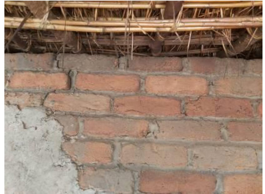
Missing wall plate for even distribution of load on the wall
