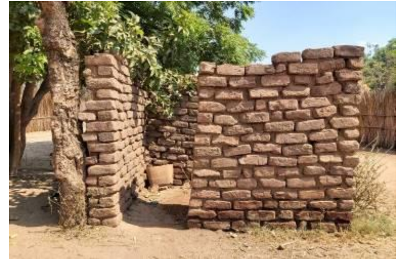
Bathroom built close to a tree and without roof
