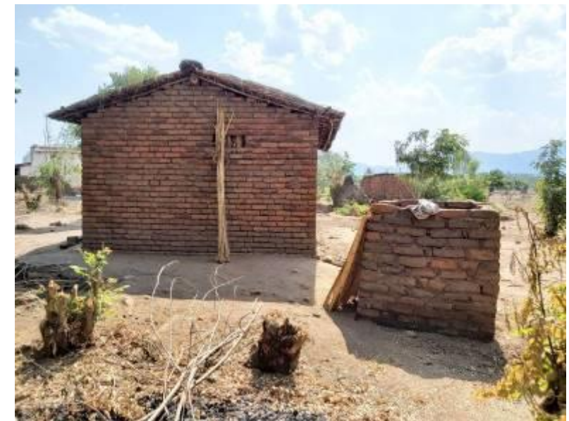
A bathroom constructed without roofing risking failure due to exposure to rain
