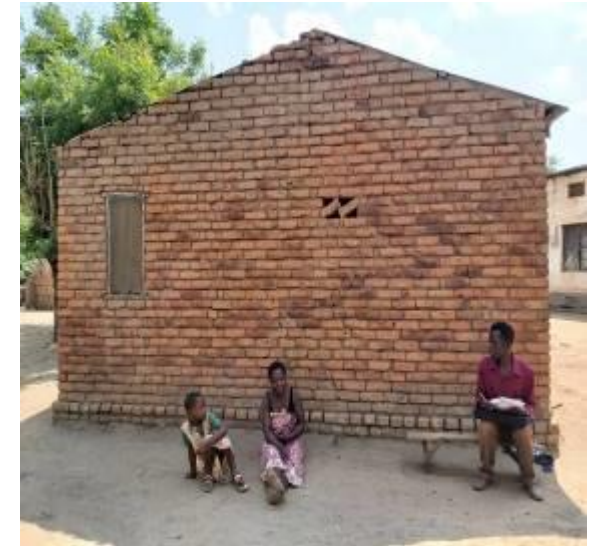
Side Gable CGI covered (burnt brick) Design – with mosquito mesh on a window
