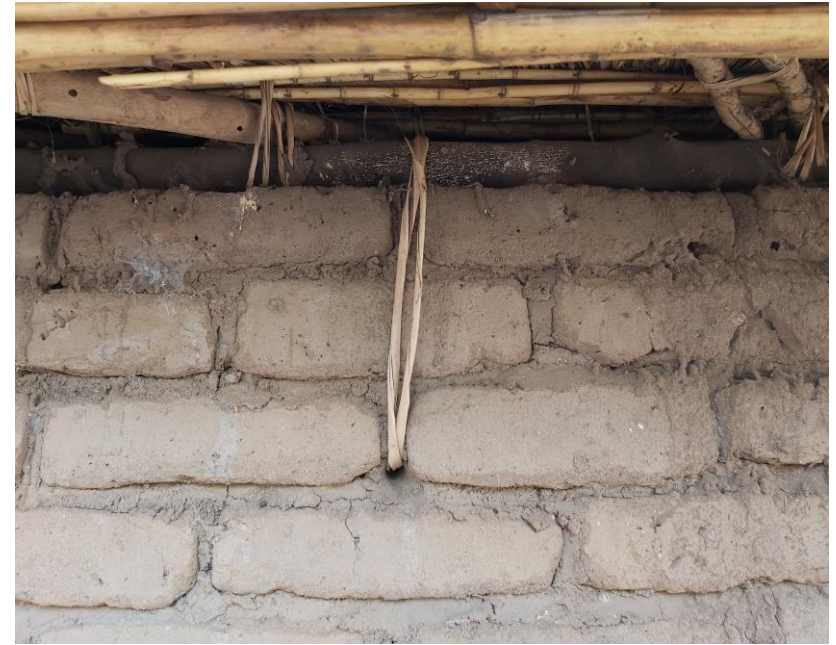
Wall-plate tied to the wall with a rope
