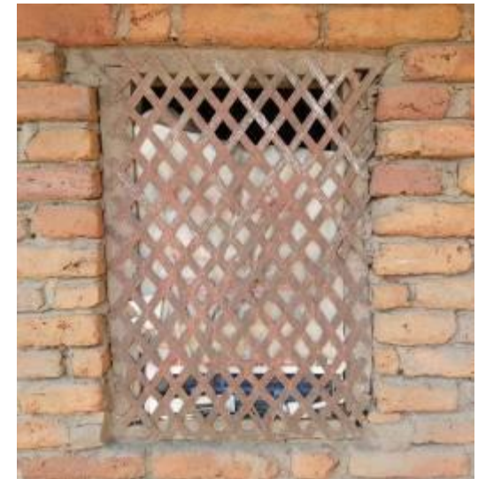
Window opening covered with steel
