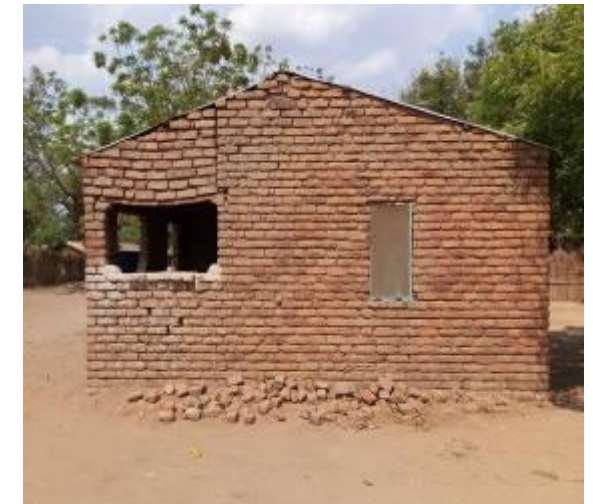
Side Gable CGI covered (burnt brick) Design – lintel failing due to heavy brick
