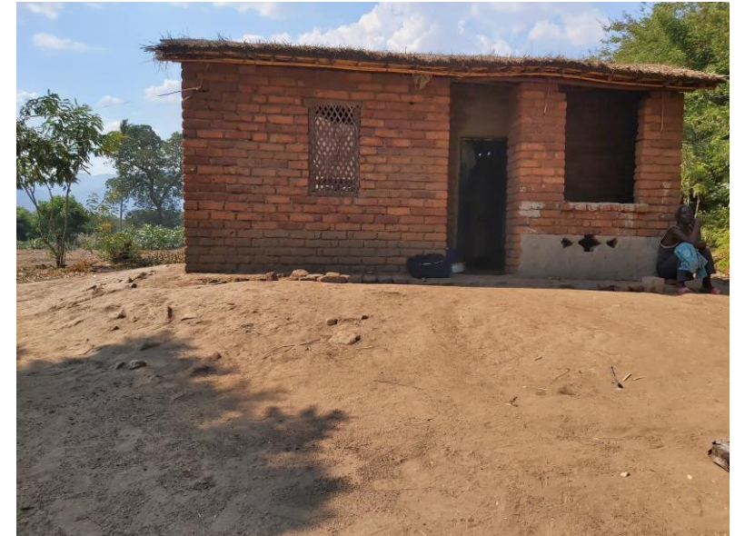
Side Gabled Grass Thatched Design – built on a raised land
