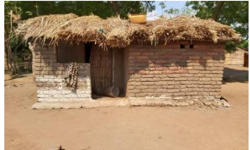
House without foundation and loose grass bundles on the roof
