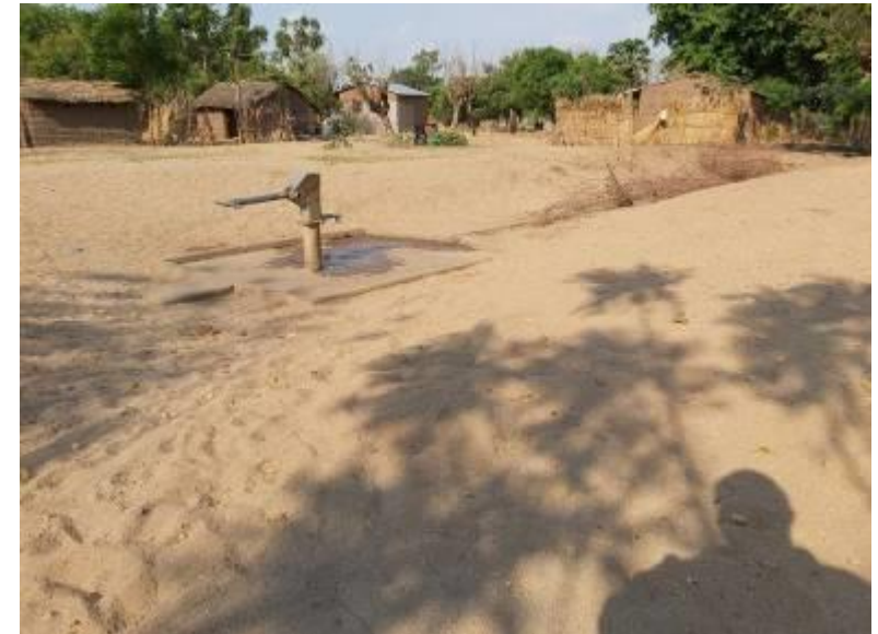
Afridev pump borehole in a heavy silted land
