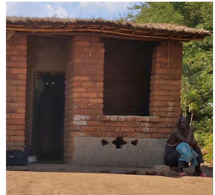
Ventilation openings on the veranda wall to help voiding the smoke
