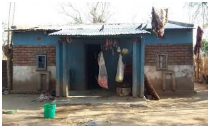
House cement-plastered up to window level with a painting finish/
