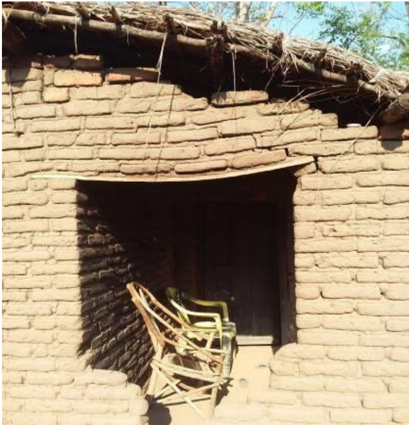
Lintel on a window opening with small thickness failing due to heavy load by bricks on top of it
