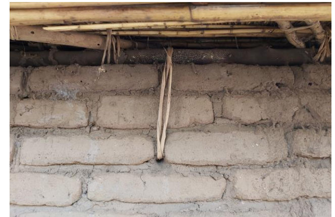
Rope binding wall plate to the wall
