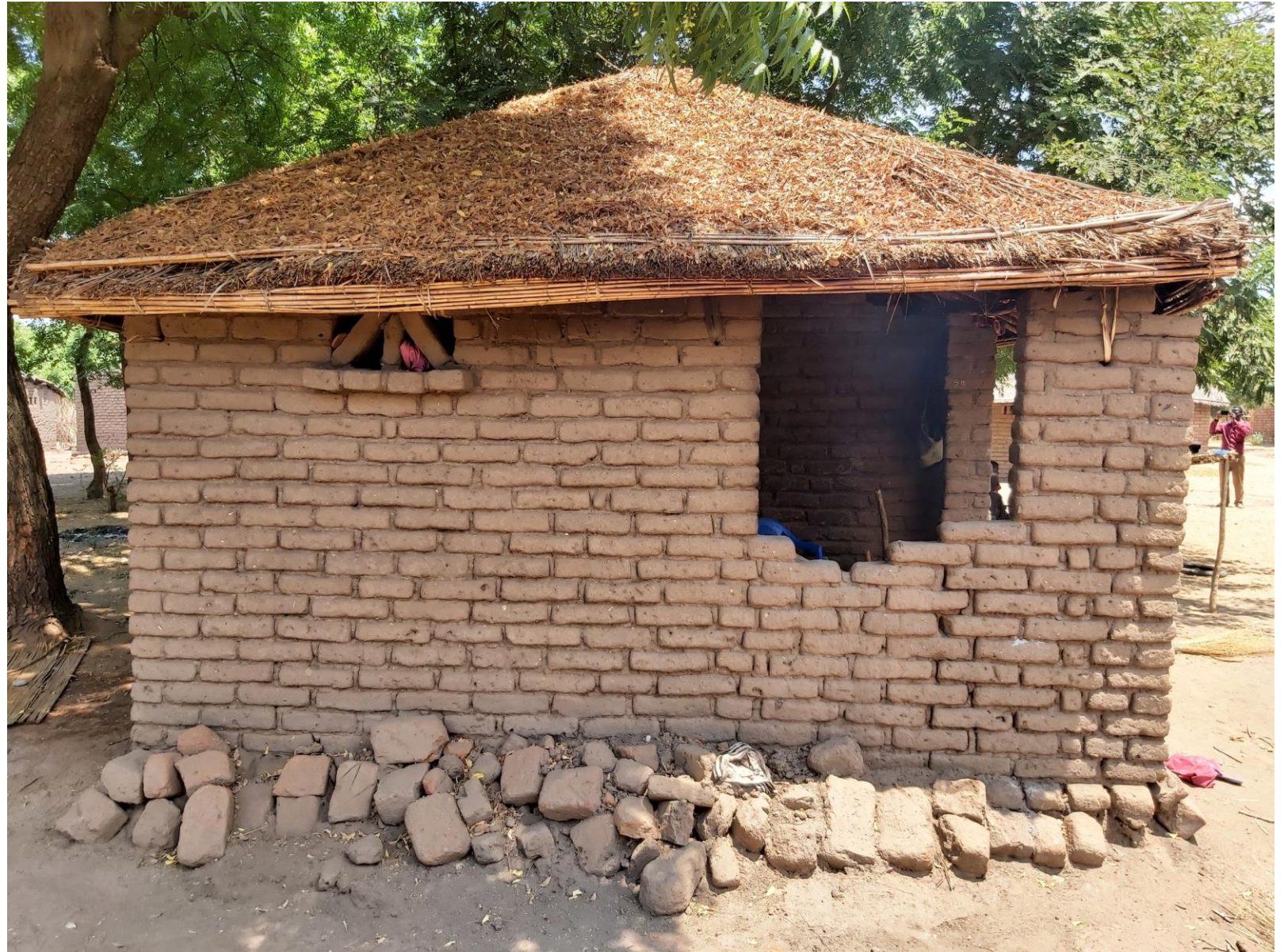
House with tied grass on a roof and an embarkment around the house
