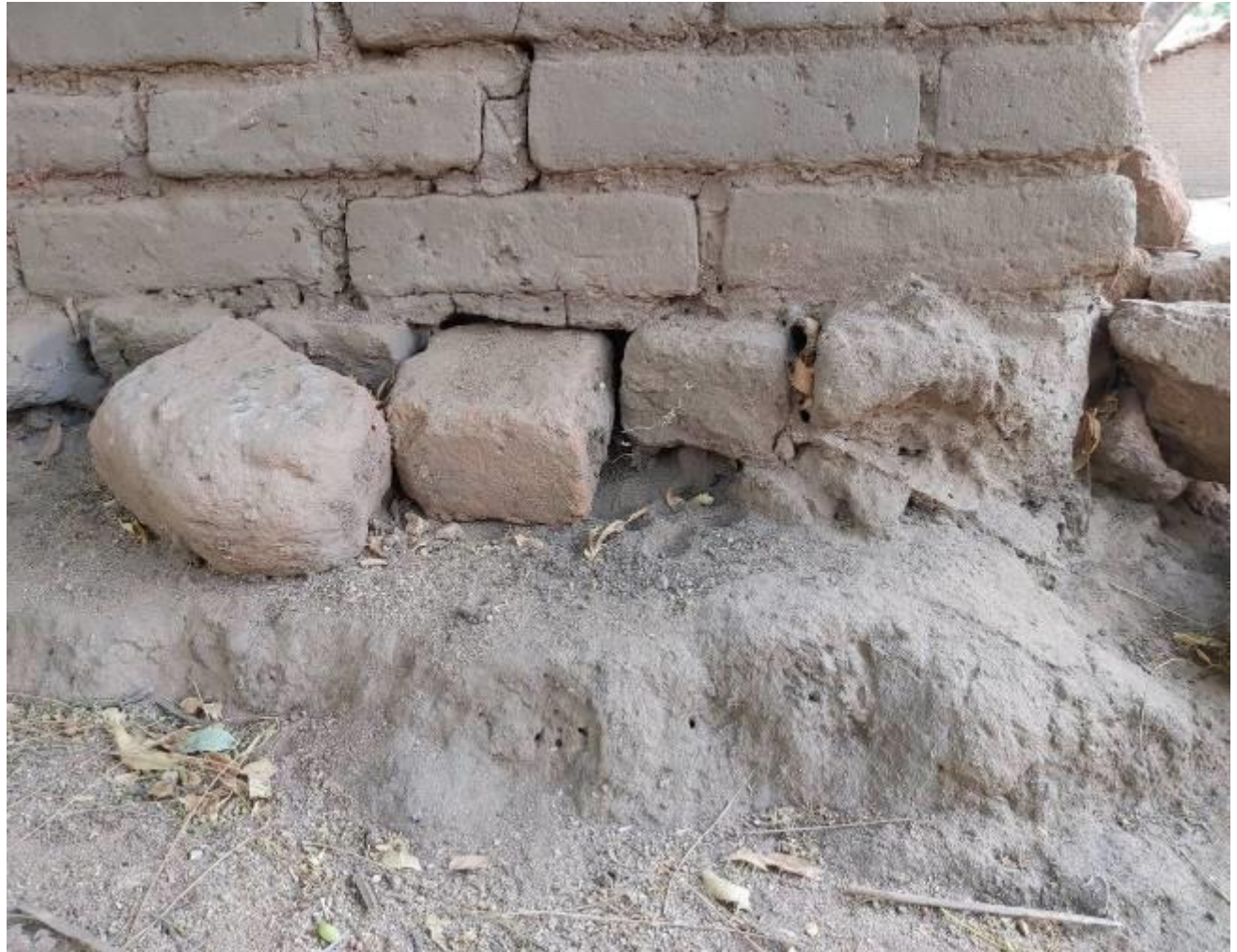
Wall starting on a header course on the ground without foundation
