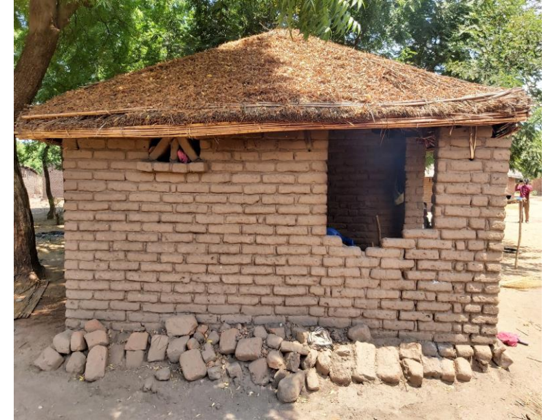
Heap (grass thatched) roof design house in the village – Side view
